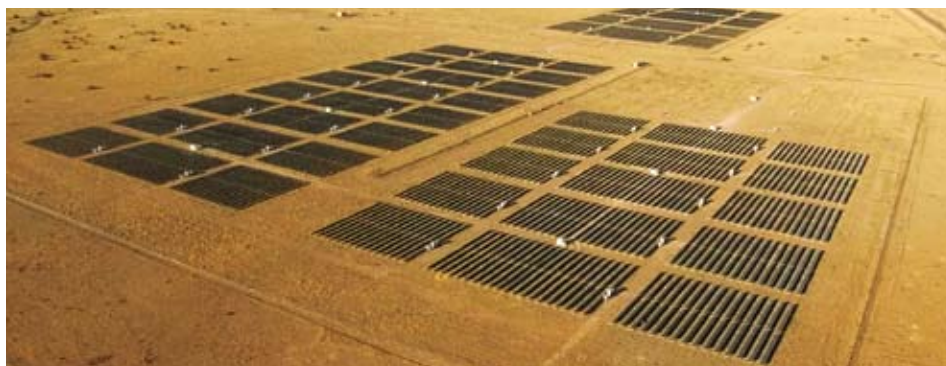
Figure 4. Springerville Generating Station in Springerville, Arizona. Credit: Tucson Electric Power
